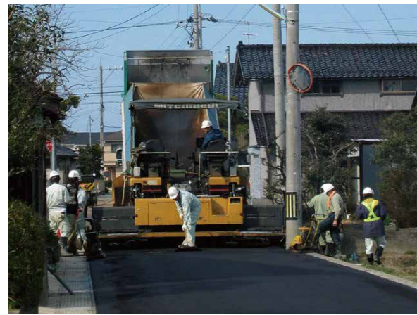
Photo-2 Capping oil-contaminated soil with asphalt pavement 12)
