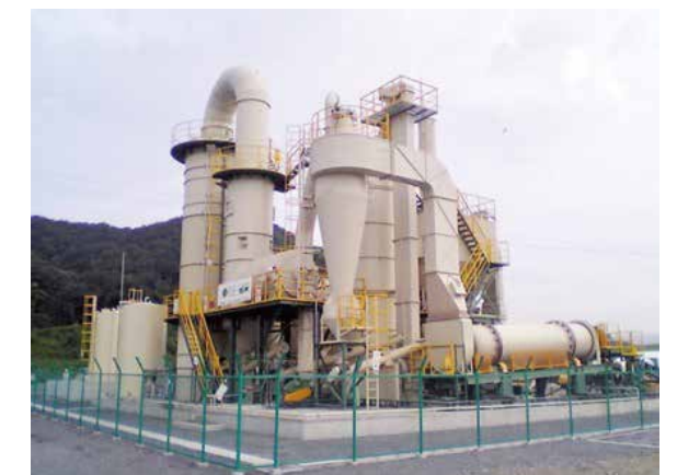
Photo-6 General view of NTR-Stage III plant
