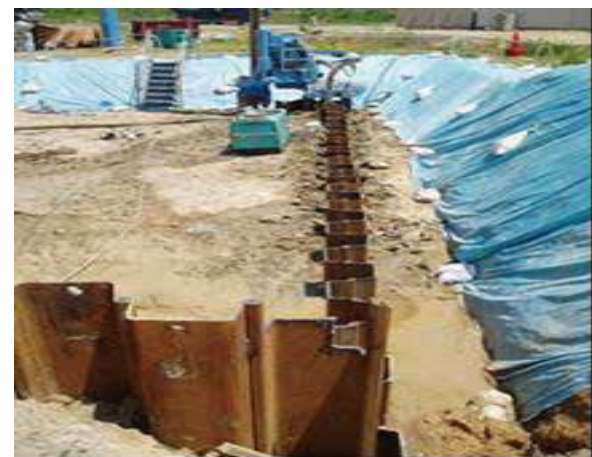
Photo-3 Cut-off wall (water barrier wall) 1)
