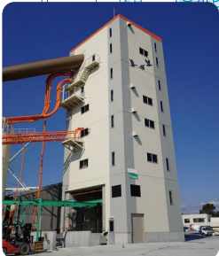
Concrete plant (BP-Related Business)
