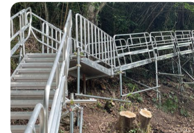
Temporary construction equipment (Other Business)
