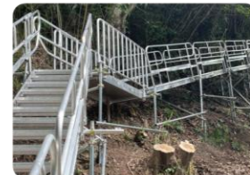
Temporary construction equipment (Other Business)
