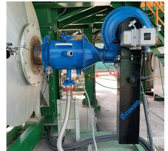
Photo 1 Hydrogen Burner
