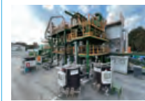
Manufactured asphalt mixtures using a hydrogen burner and conducted trial paving (2023)
