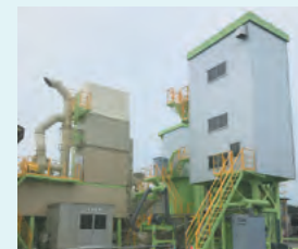
A plaster-based solidification material manufacturing facility A plant facility which manufactures gypsum hemihydrate from dried gypsum powder, which is blended with cement and lime to manufacture solidification material.
