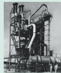
1958: Nikko's first asphalt plant completed
