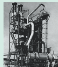
1958: Nikko's first asphalt plant completed
