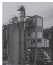
Developed compact concrete plants (1979)
